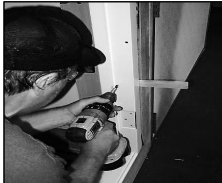
Shim and fasten with provided 3½" deck screws
