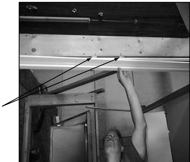
Readjust to square the frame if the difference between A & B is greater than 1/16" (1.5 mm)
