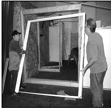
Place Frame in Rough Opening
