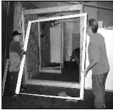
Place Frame in Rough Opening
