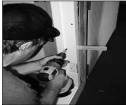
Shim and fasten with provided 3 1/2" deck screws
