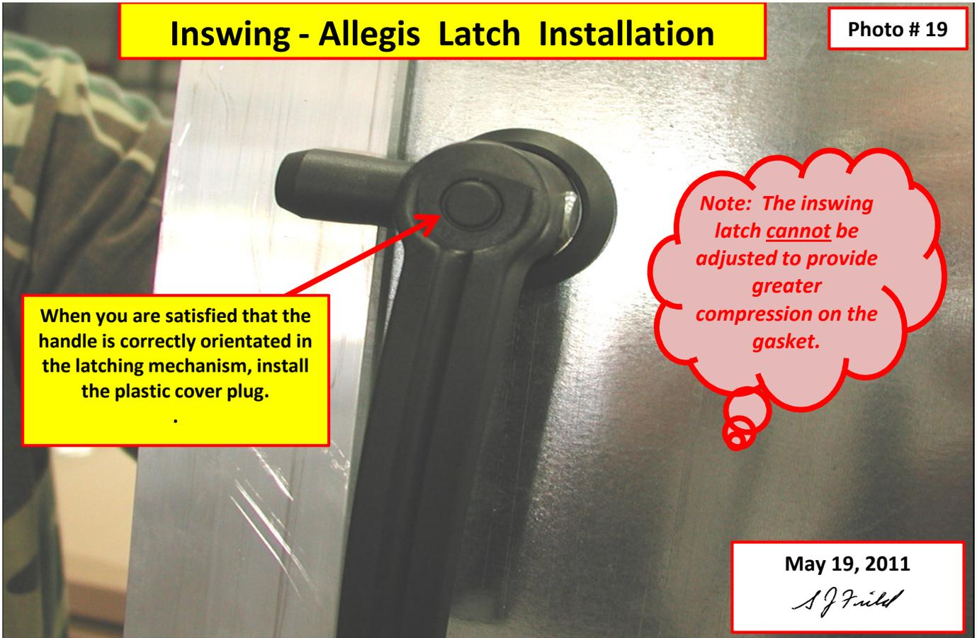
When you are satisfied that the handle is correctly orientated in the latching mechanism, install the plastic cover plug.
