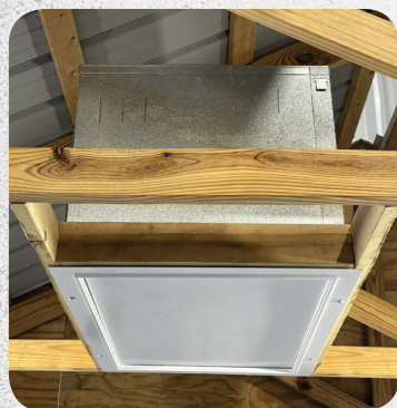
INSULATION DAM Installed with Ceiling Access Door Patent Pending
