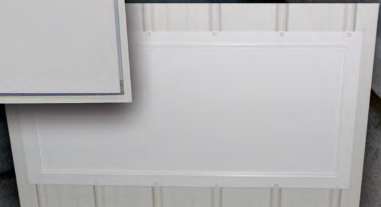
Installed Door View
