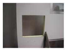
2. The view port frames are pre-sealed with foam tape applied to the underside of the trim flange. Inspect the joints of this tape prior to installation and add sealant in the corners if any gaps have appeared. (Any typical exterior grade caulk-type construction sealant will suffice.)
