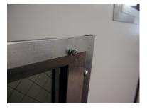
9. Tighten each screw so that the trim flange is drawn down, tightly, against the door skins.
