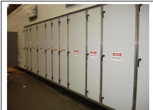
Area of Concern – Wide Angle View
