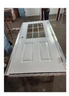
3. Run a bead of silicone along the leg to seal against the jamb. Using the supplied self-tapping screws, attach the Assembly Strip to the jamb. Be sure it is  $\frac{1}{4}$ " from the top of the door.
