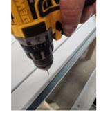
2. Set the assembly strip onto the jamb, ¼" from the top of the door and mark your holes. Pre-drill pilot holes.
